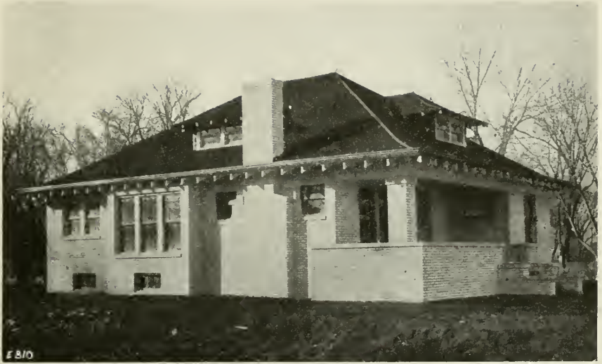
FIG. 125.—BUNGALOW OF CONCRETE BRICKS.
